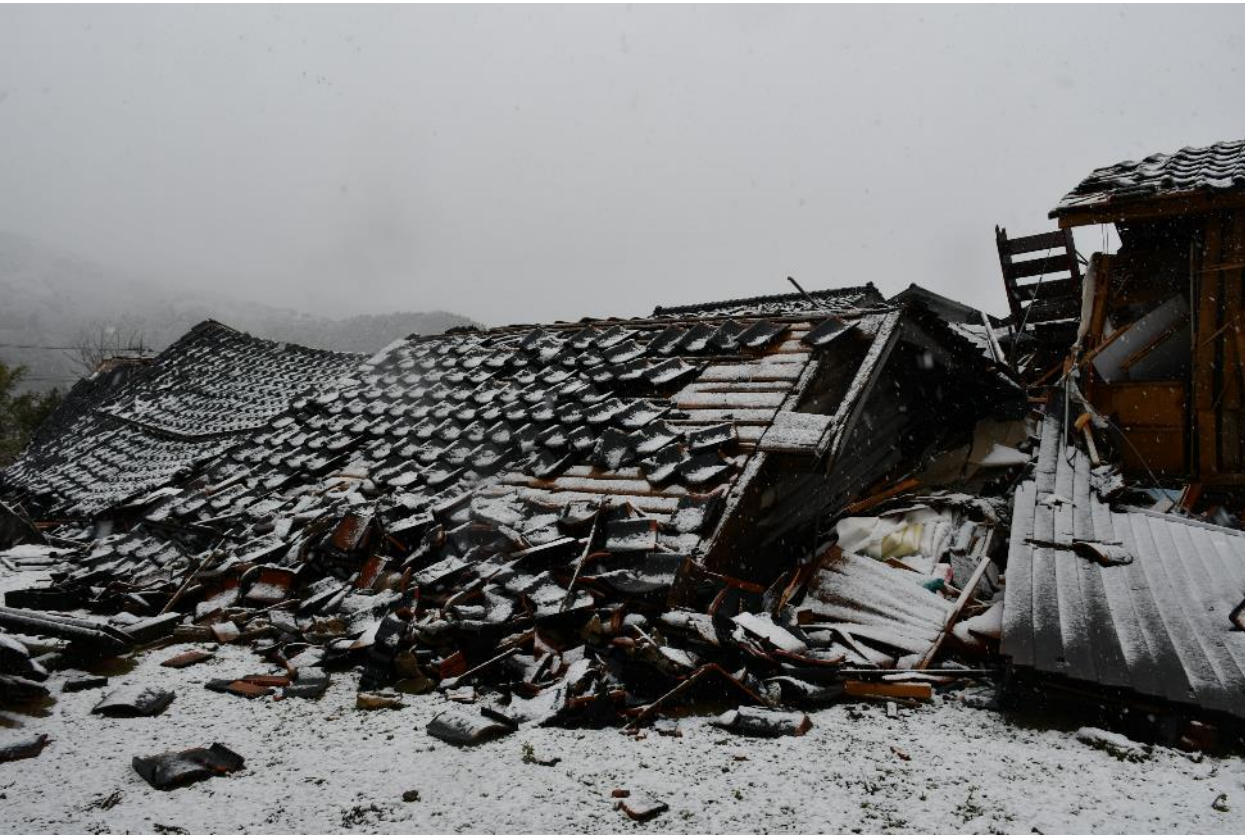
Collapse of wooden houses (Map①)
