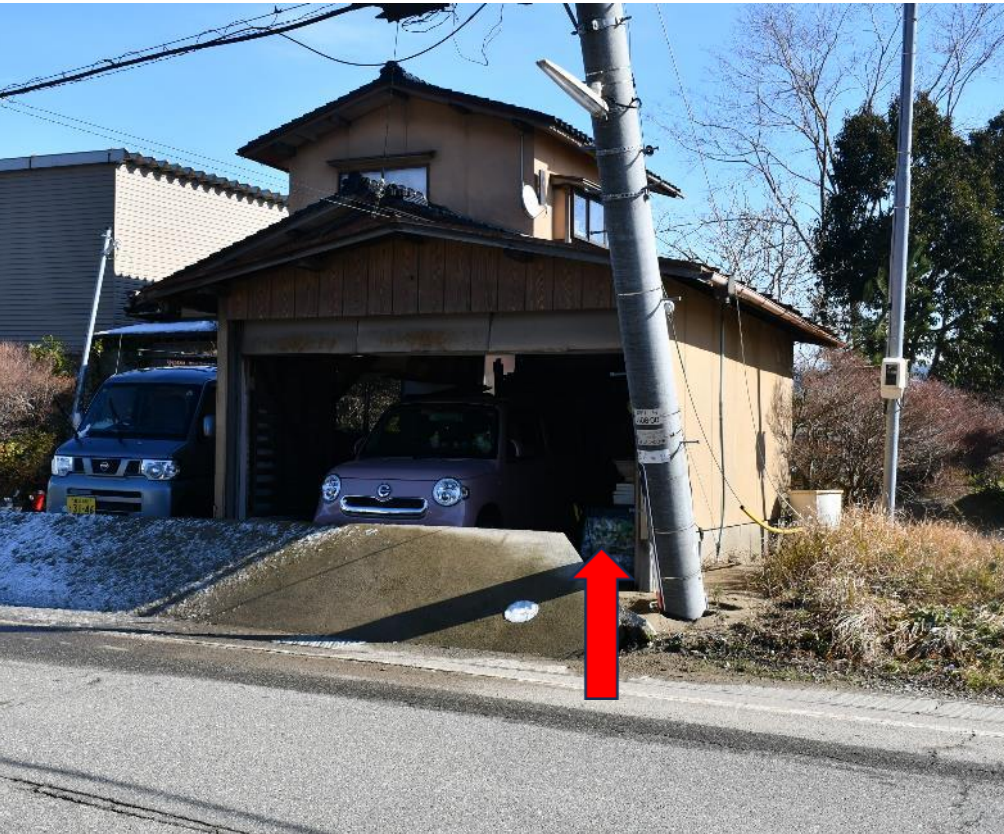
Lateral flow of liquefied ground in the dunes hinterland (Map③)
