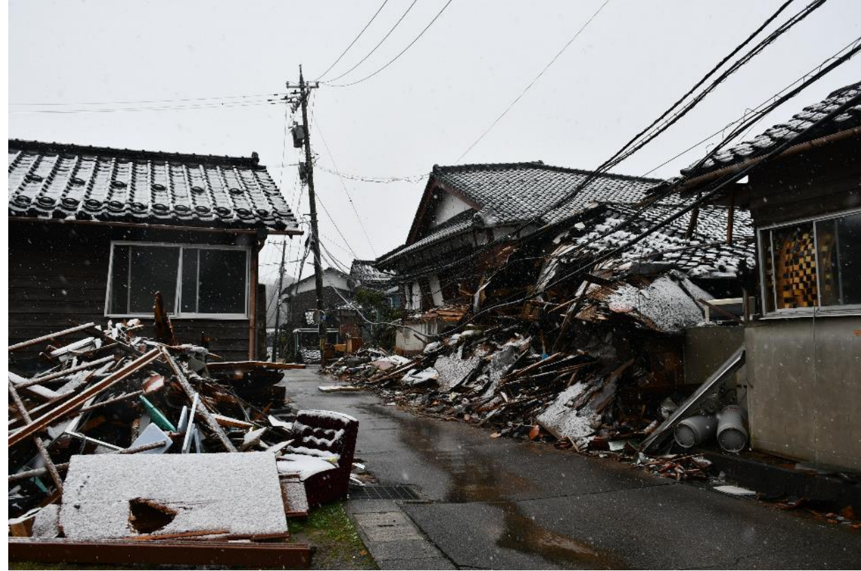
Collapse of wooden houses (Map①)
