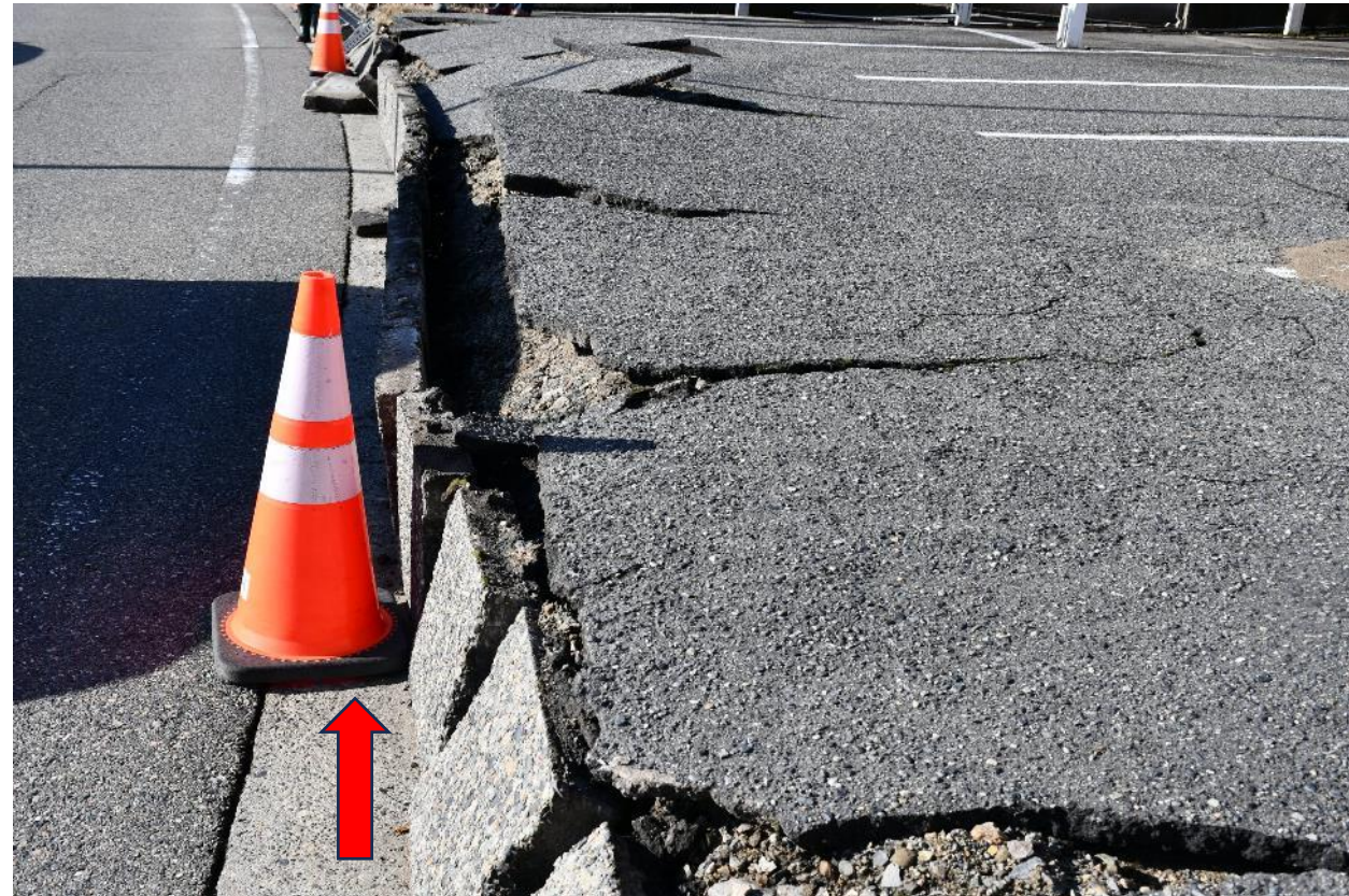
Uplift of the ground due to lateral flow (Map①)
