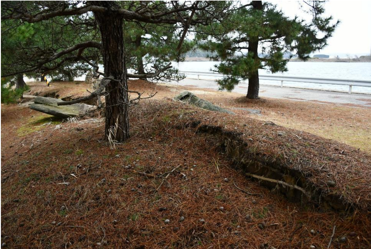
Uplift and depression of the ground due to lateral flow of liquefied ground (Map②)
