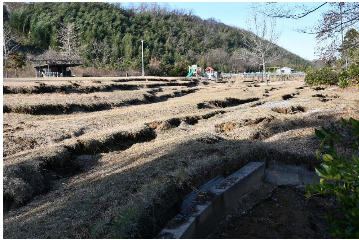
Ground deformation due to lateral flow (Map①)
