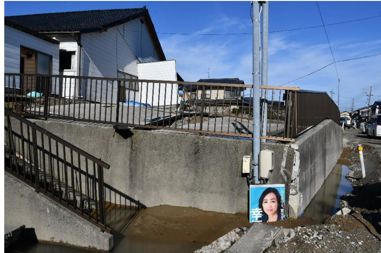
Lateral flow of liquefied ground in the dunes hinterland (Map③)
