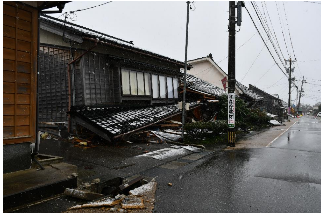
Collapse of wooden houses (Map①)
