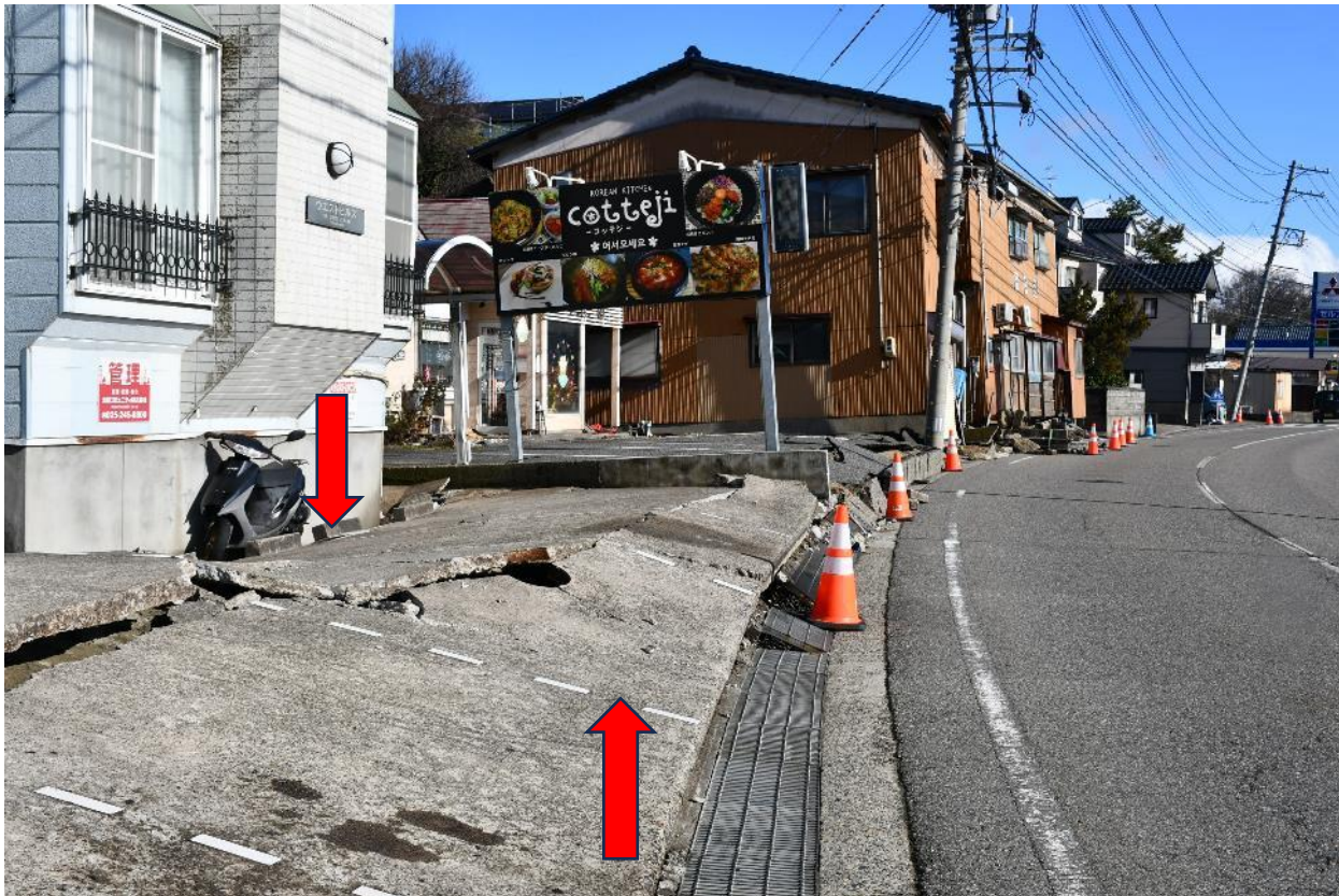
Uplift of the ground due to lateral flow (Map①)
