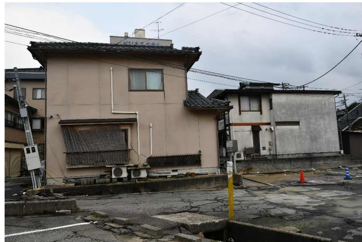
Inclination of the buildings in front of Wakura Onsen Station due to liquefaction (Map⑤)
