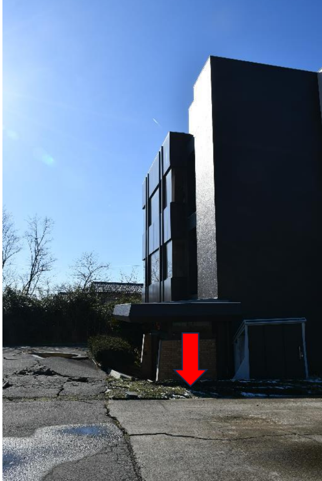
Subsidence of RC building due to liquefaction (Map②)
