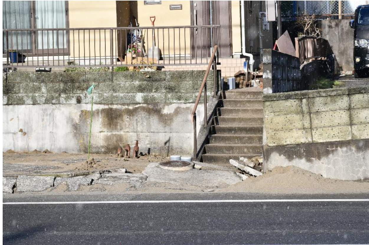
Lateral flow of liquefied ground in the dunes hinterland (Map①)
