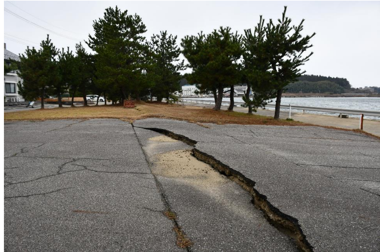
Uplift and depression of the ground due to lateral flow of liquefied ground (Map②)
