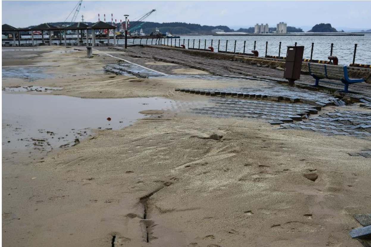
Subsidence and ejected sand due to liquefaction (Map④)
