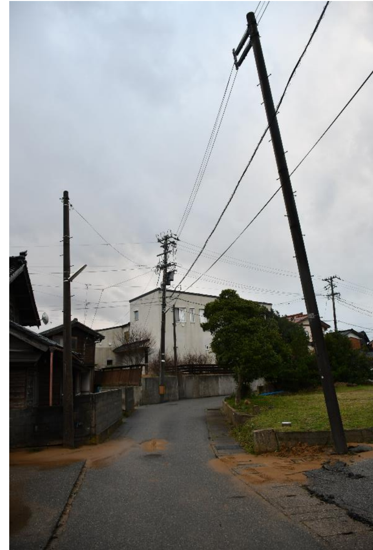
Subsidence of houses, utility poles due to liquefaction (Map①)
