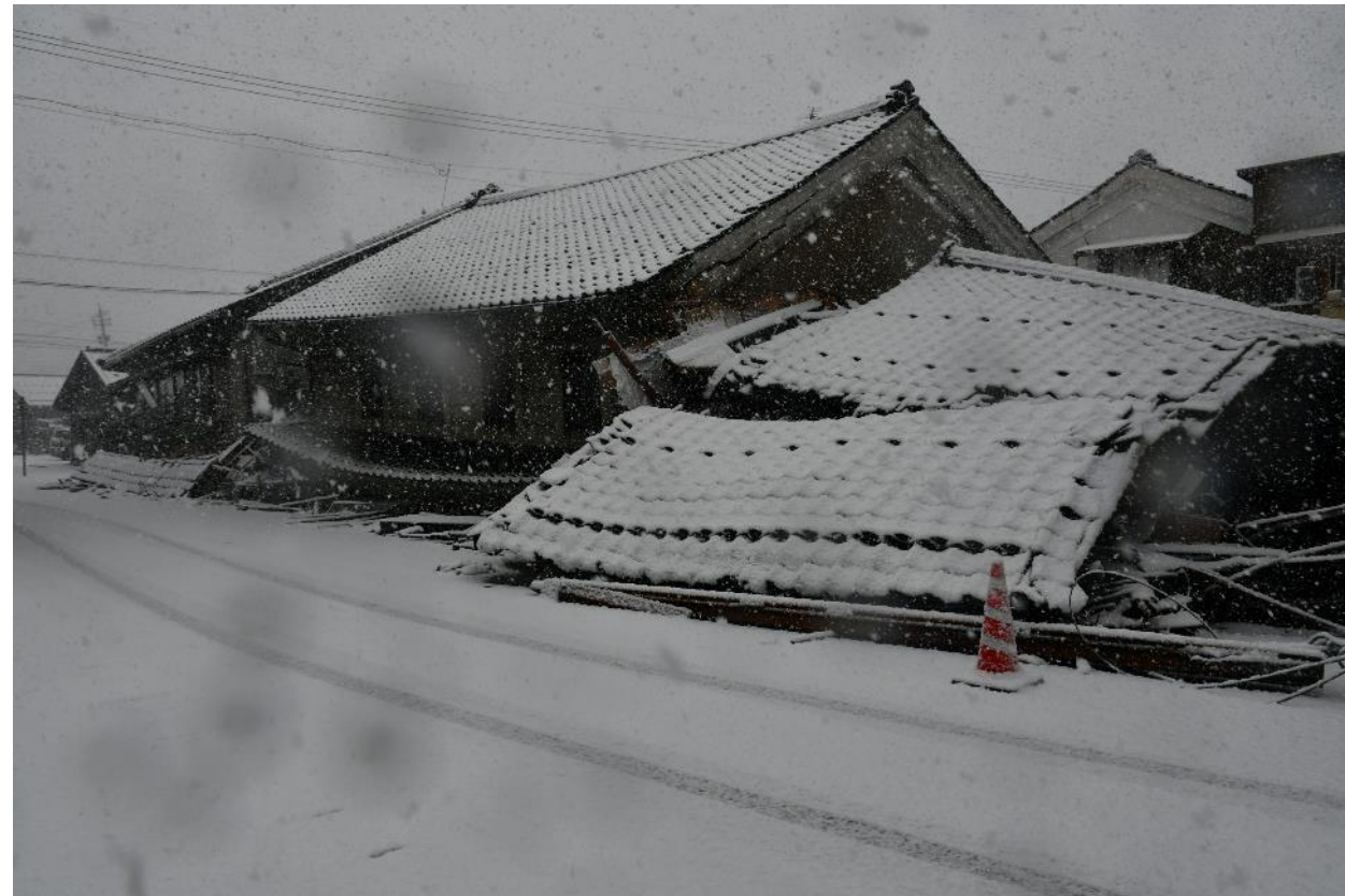
Collapse of wooden house (Map③)
