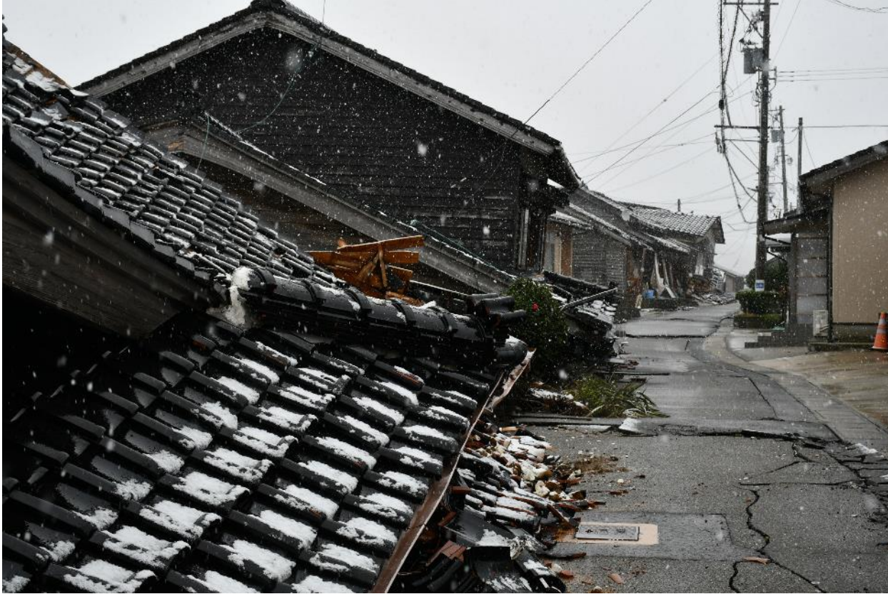
Collapse of wooden houses (Map①)
