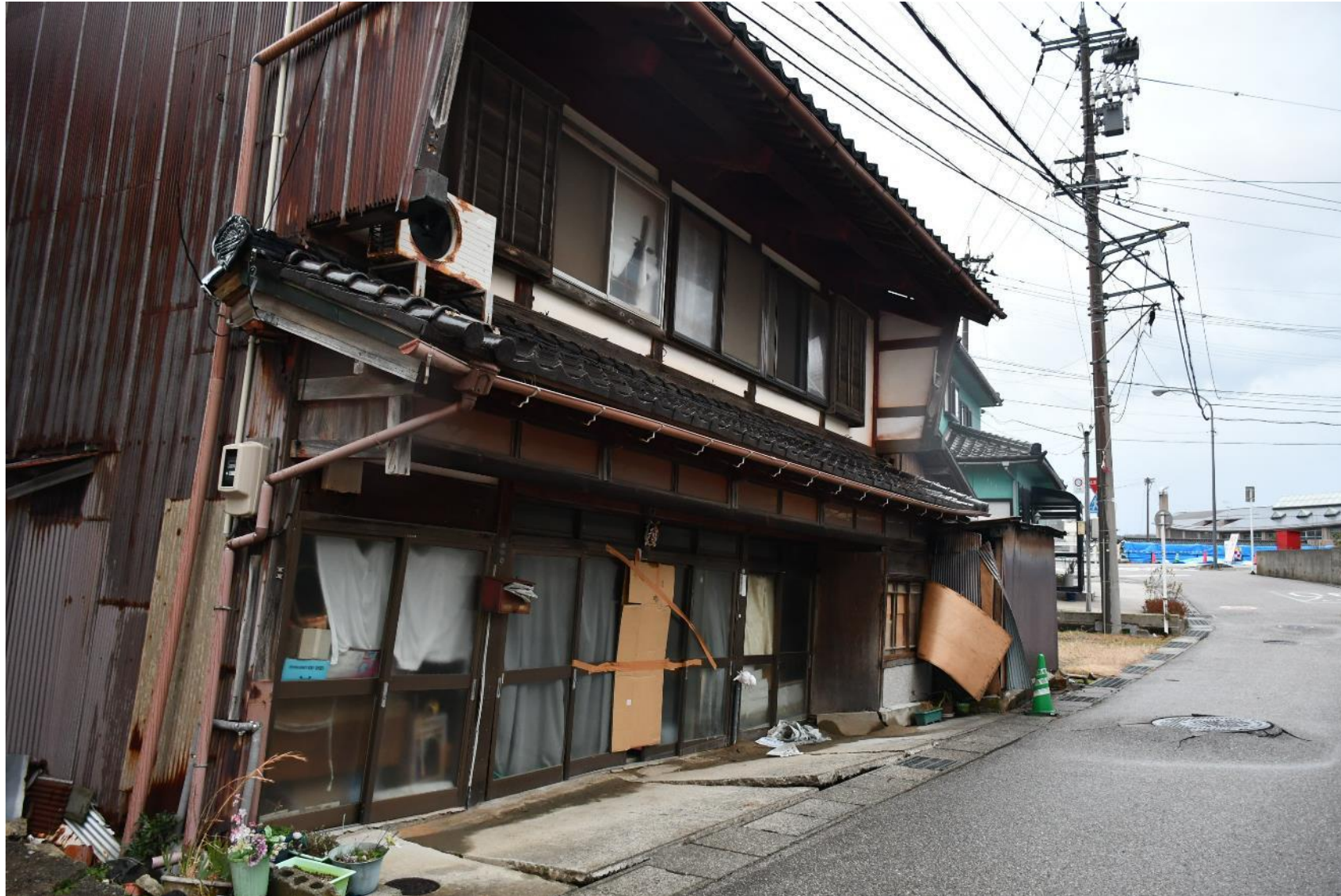
Subsidence of houses, utility poles due to liquefaction (Map①)
