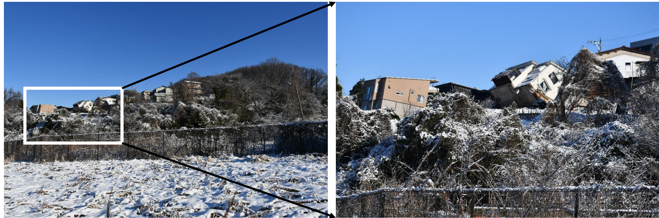
Damage to houses caused by landslides on embankment of developed residential areas (Map①)
