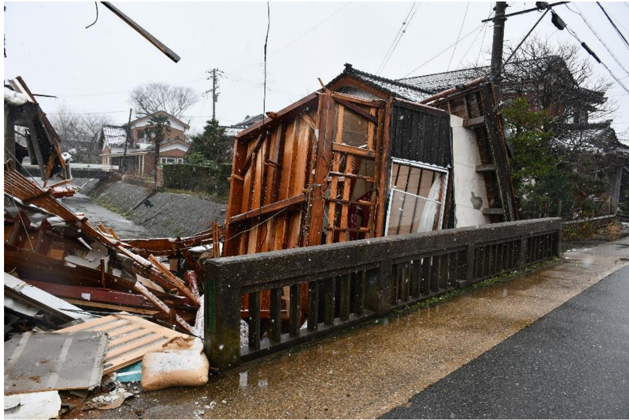
Collapse of wooden houses (Map①)
