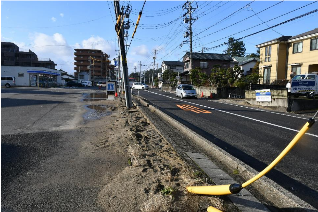
Lateral flow of liquefied ground in the dunes hinterland (Map①)
