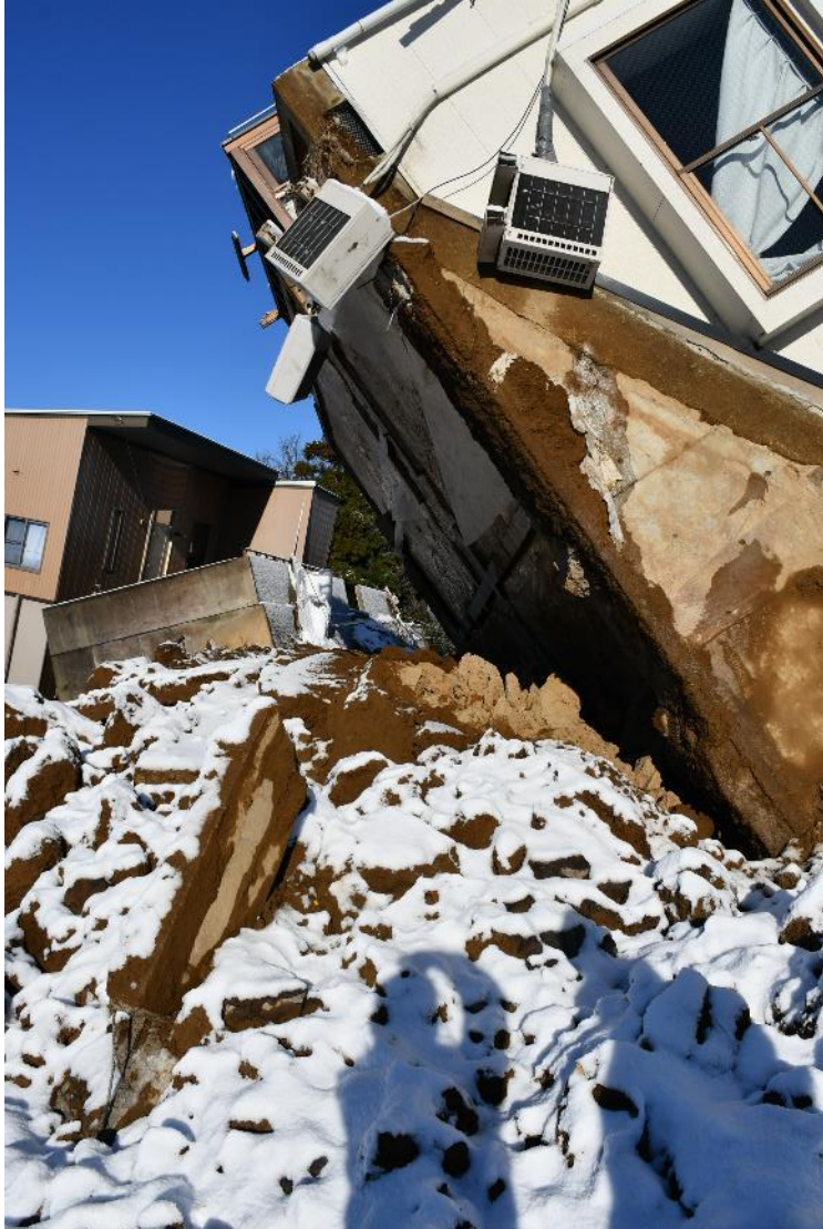
Damage to houses caused by landslides on embankment of developed residential areas (Map①)
