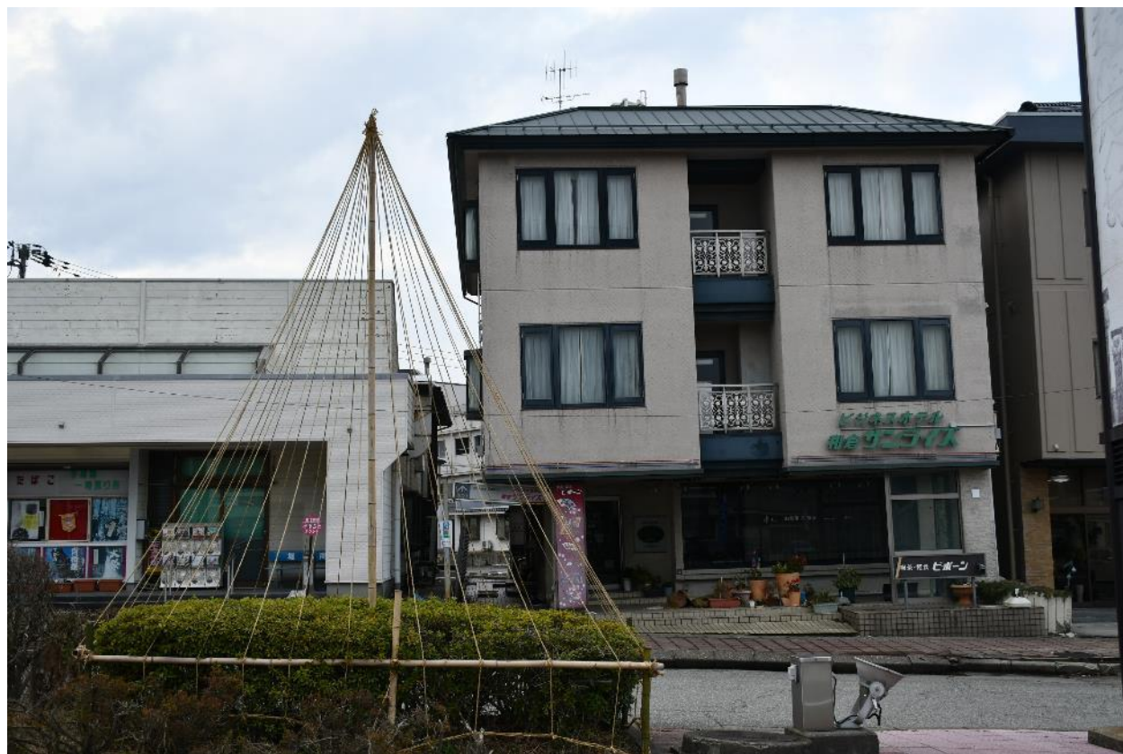
Inclination of the buildings in front of Wakura Onsen Station due to liquefaction (Map⑤)
